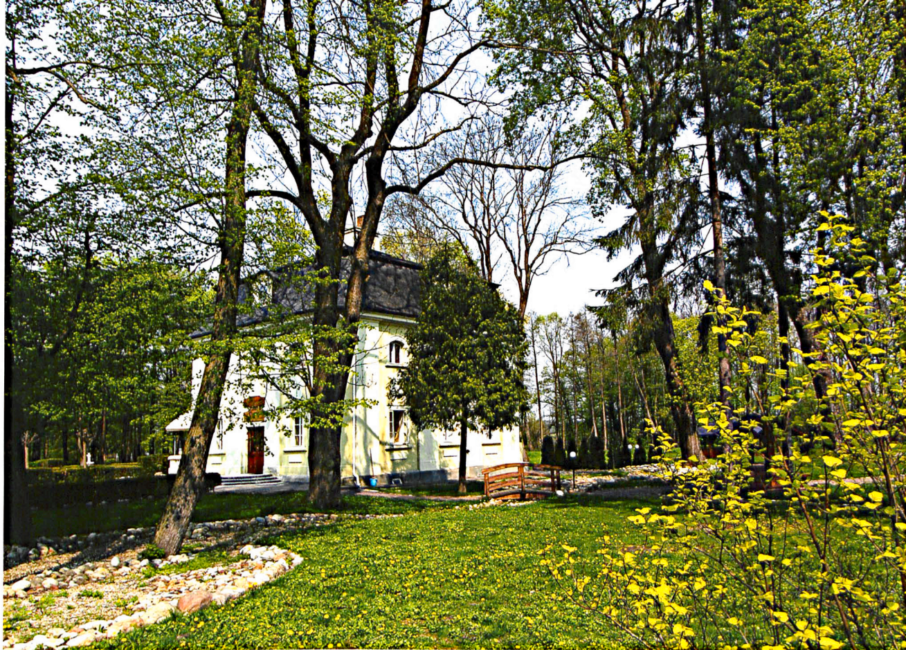
W dawnym parku pałacowym w Sosnowicy. Former palace park in Sosnowica.
